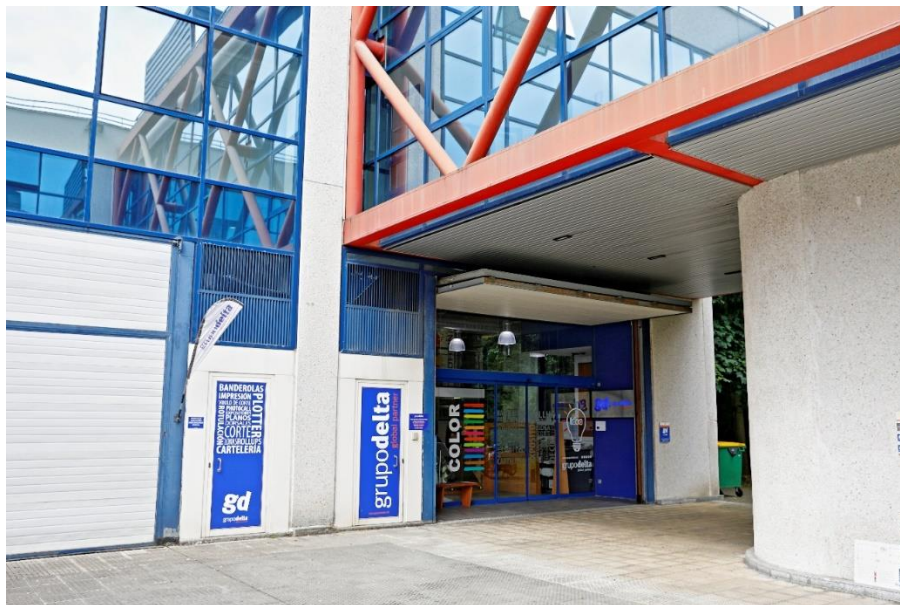
Fig. 1. Grupo Delta's current facilities in Zuatzu
